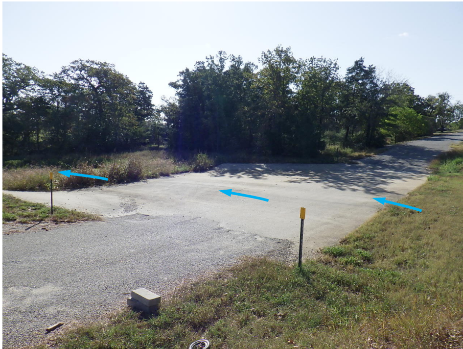
Photo 16. View of the spillway channel/roadway crossing approximately 320-feet downstream from the spillway inlet. The direction of flow is noted by the arrow.
