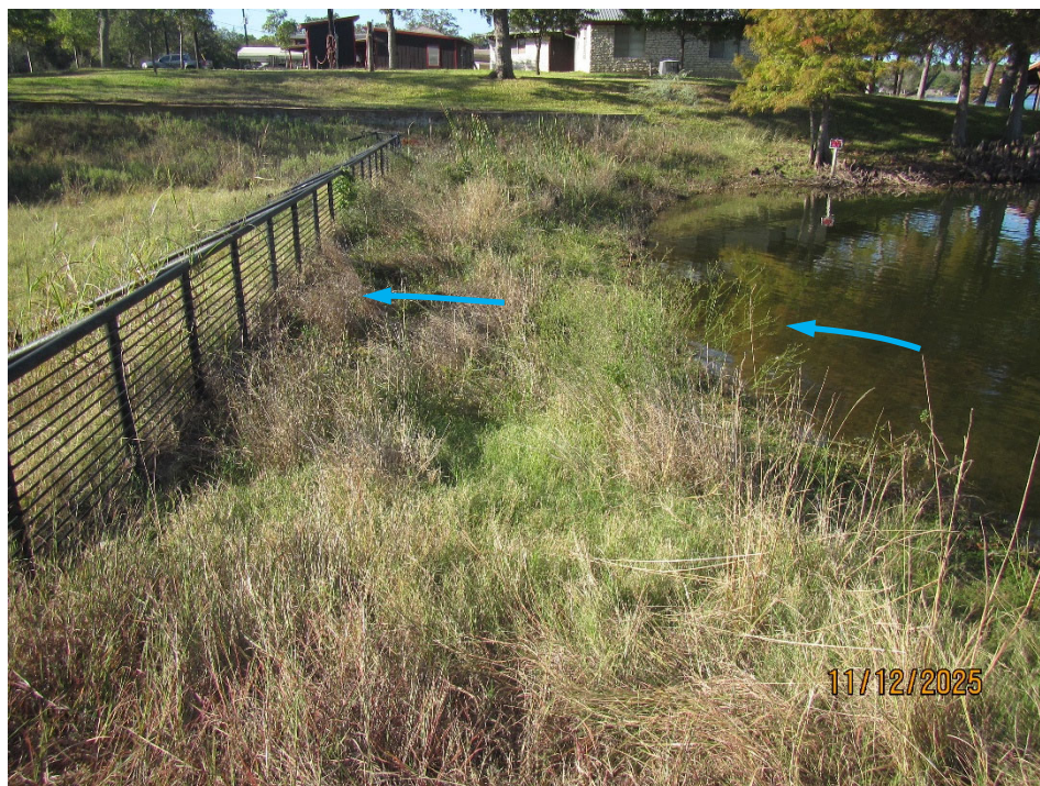
Photo 14. View of the spillway inlet looking right from the left end of the spillway channel. Note the tall grass growth along the inlet just upstream of the debris guard fence. The direction of flow is noted by the arrows.
