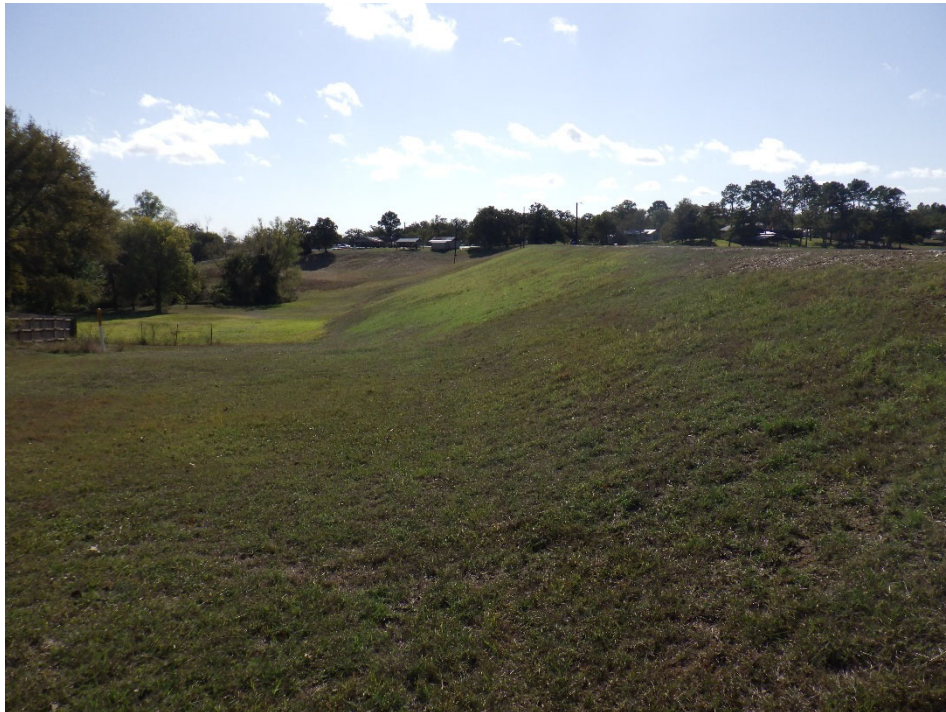
Photo 8. View of the downstream slope looking right from the near left end of the dam. Note the well-maintained grass cover.
