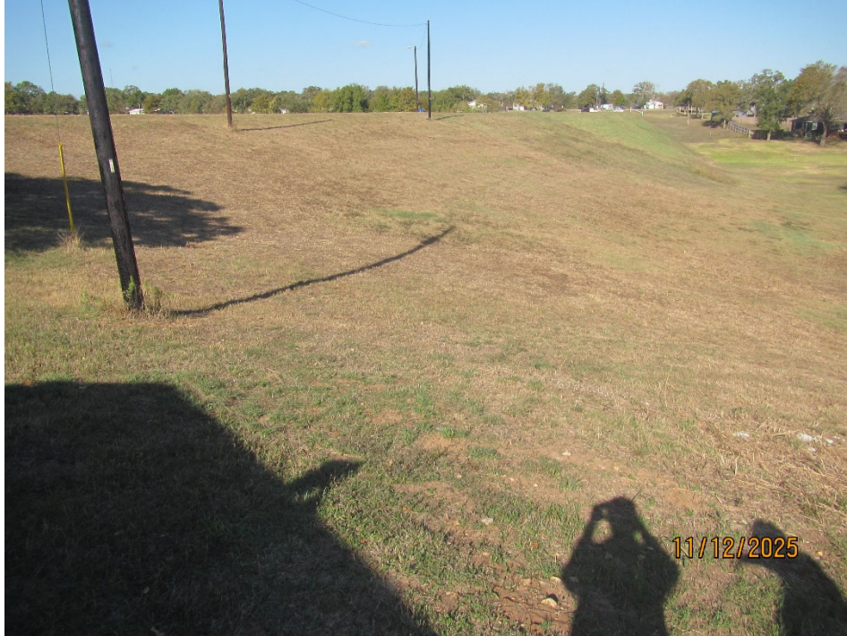
Photo 9. View of the downstream slope looking left from the right end of the dam. Note the well-maintained grass cover along the previously noted damaged areas.
