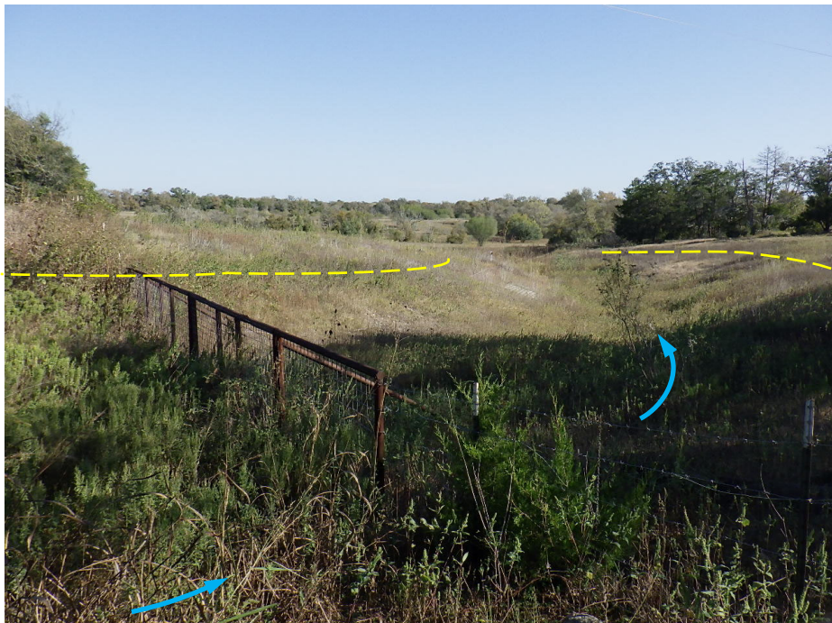
Photo 18. View of the downstream channel looking downstream from the spillway channel/roadway crossing. Note the brush and grass growth along the fence traversing the spillway channel. The direction of flow is noted by the arrows.
