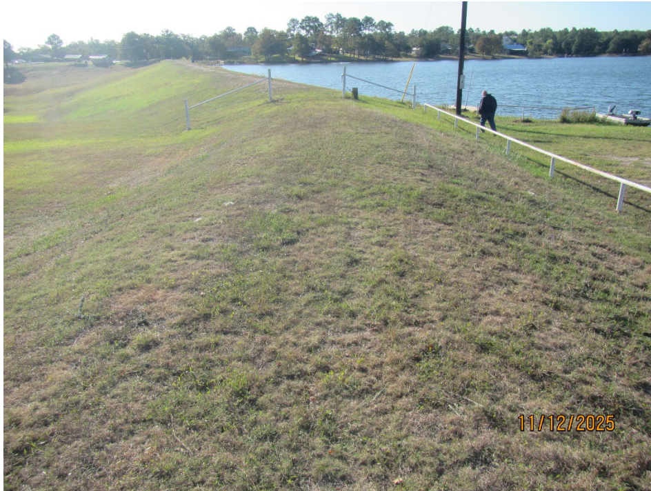
Photo 1. View of the crest looking right from the left end of the dam. Note the well-maintained grass cover.
