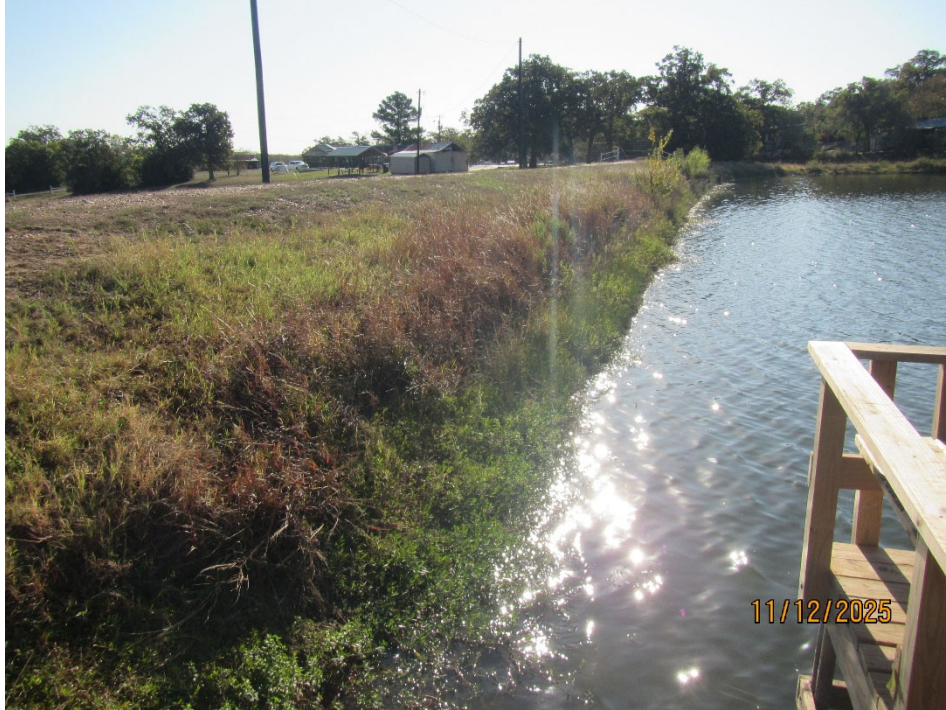
Photo 5. View of the upstream slope looking right from the middle of the dam. Note the taller grass growth along the right end of the slope.
