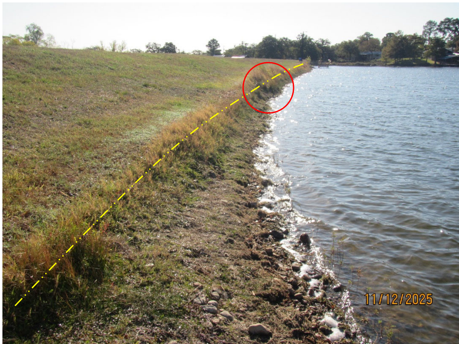
Photo 4. View of the upstream slope looking right from the near left end of the dam. Note the slight uneven shoreline (circled) and taller vegetative growth along the approximate normal pool level (dashed line).
